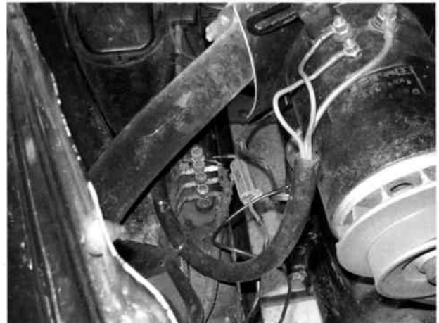
Photo graph 11 - the resistor unit in position
