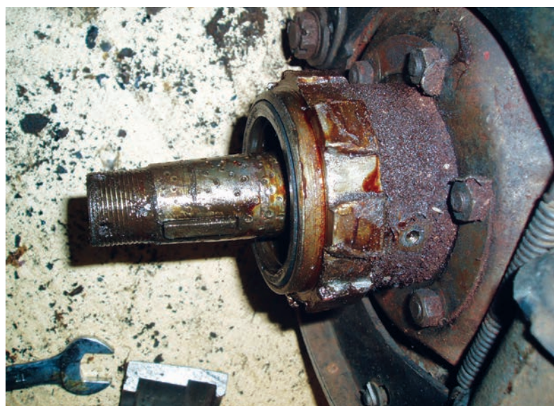
TL : photograph 2 - it is essential to reduce the width of the spacer between the bearings by 2mm. TR : photograph 3 - protruding bearing because the width of the spacer has not been reduced CL : photograph 4 - drum taper damaged through use with incorrectly fitted wheel bearings CR : photograph 5 - temporary remedy is to raise a series of 'dinks' on the driveshaft BR : photograph 6 - 'dinked' driveshaft ready to refit damaged drum taper as a temporary repair
