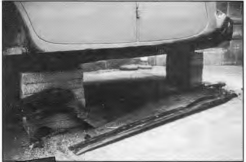
Outer sill and strengthening steel removed, exposing severe rust and damage to inner sill caused by the fitting of the strengthening steel, which must have been removed from a lorry chassis.
