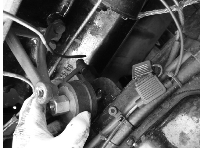
Photo 5 - fitting the silentbloc unit
