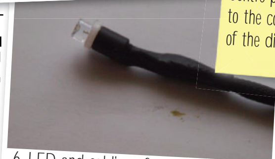
6. LED and cabling after sealing with heat shrink tubing.
