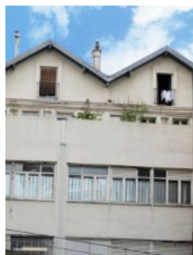
Built on the flat roof of the depot
