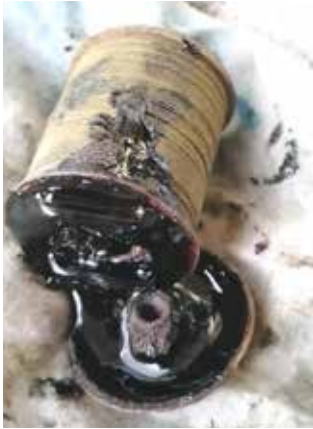
Crushed pickup pipe Tubing (right)
