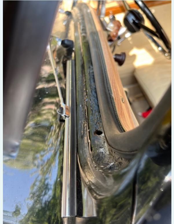
Picture 4 Internal seal fitted
