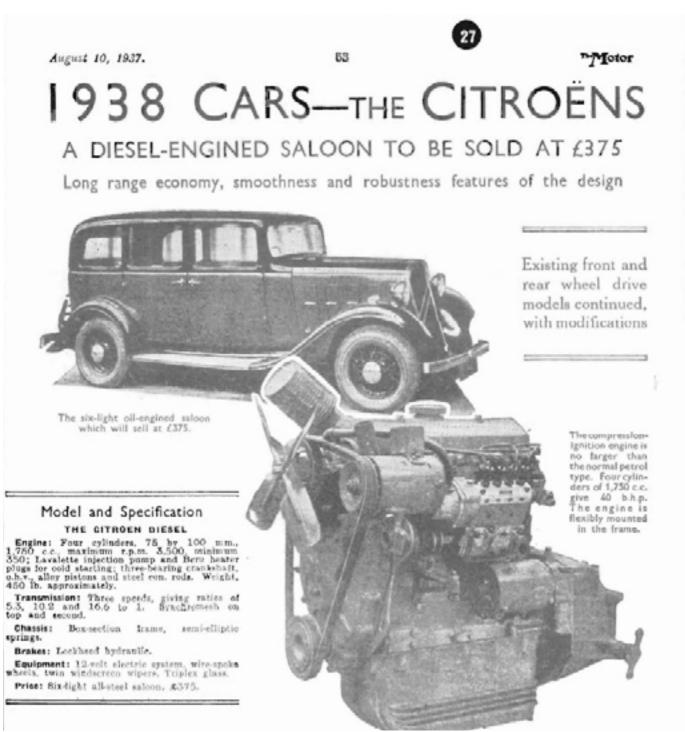
Citroen in common with many European manufacturers had a legacy of diesel cars and so it would be logical, given a similar mechanical layout, that there would be experiments carried out converting Tractions to Diesel, or Heavy Oil as DVLA like to term it. RWD Rosalies were certainly offered in the late 1930's with a diesel engine. It is also believed that some experiments were undertaken by Citroen with a diesel powered Traction, but none ever found their way into production. (cont,d.)
